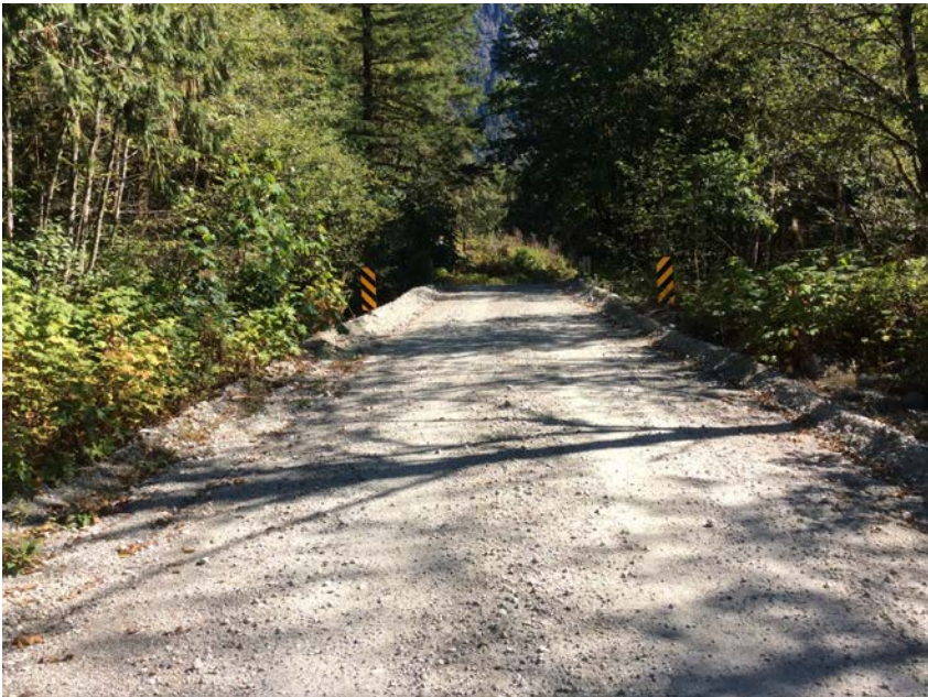
Approach from Right Bank when facing downstream
