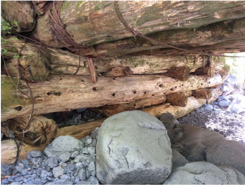
Left Bank Abutment when facing downstream
