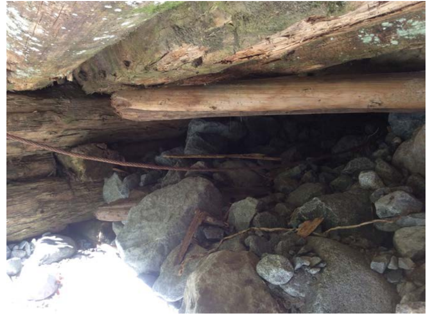
Right Bank Abutment when facing downstream
